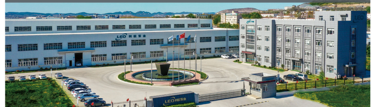
Pump Manufacturing Base for Petrochemical Industry
